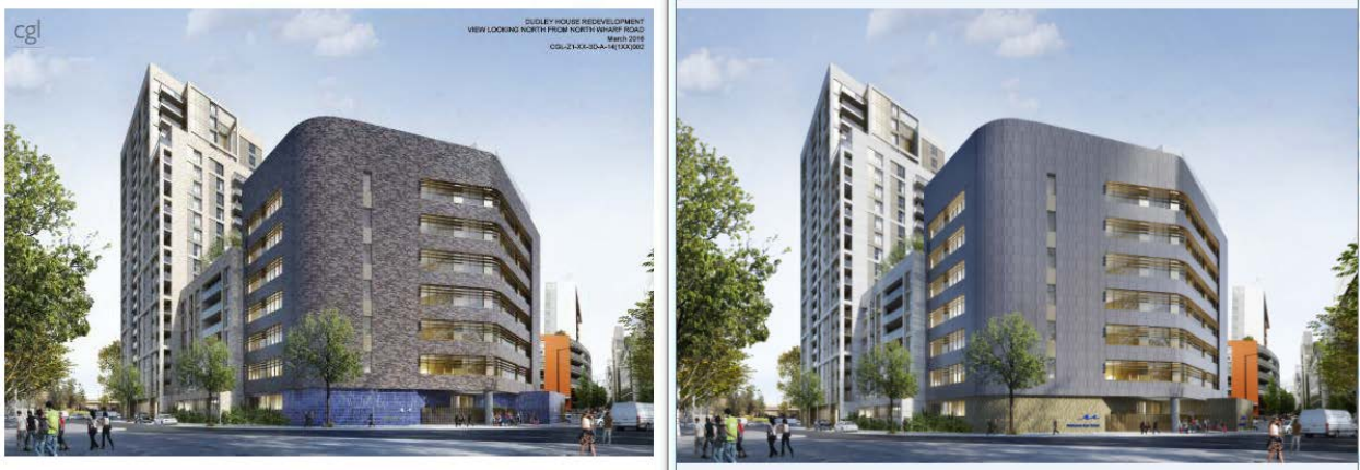
As approved scheme (left) with brick slip cladding and as now proposed with terracotta cladding (right).
