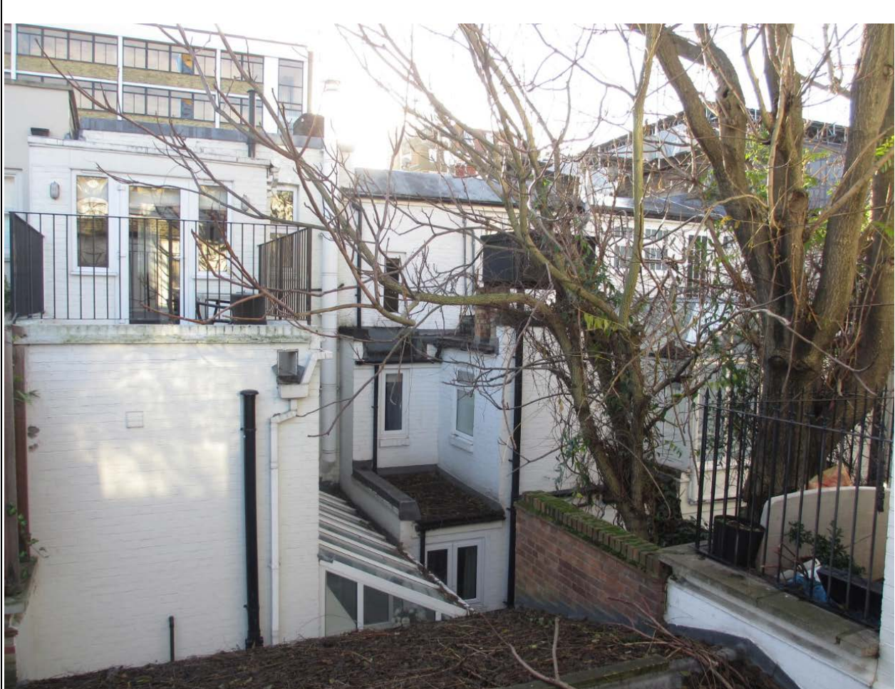
View from first floor of No. 10 Fairholt Street looking towards Nos. 32 and 34 Cheval Place (tree in adjacent garden of No. 9 Fairholt Street has since been felled).
